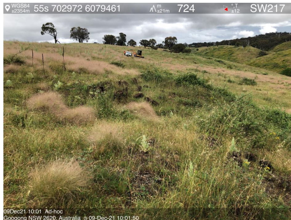
Photo 2 – View of western edge of the development area. Pit 1 being excavated.
